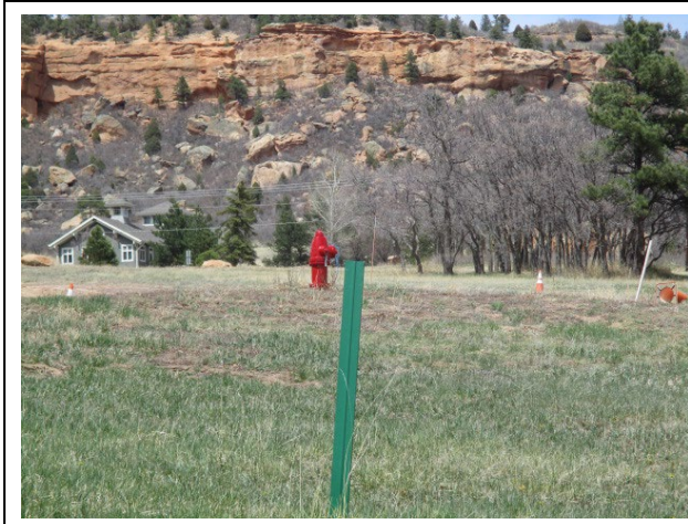
Fire Hydrant on the property
