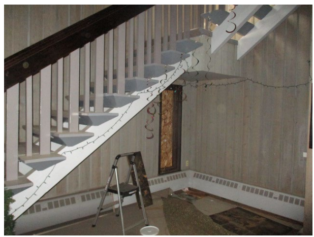
Access to crawl space
