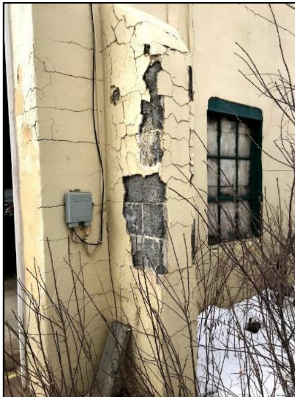
Figure 19: Exterior Deterioration
